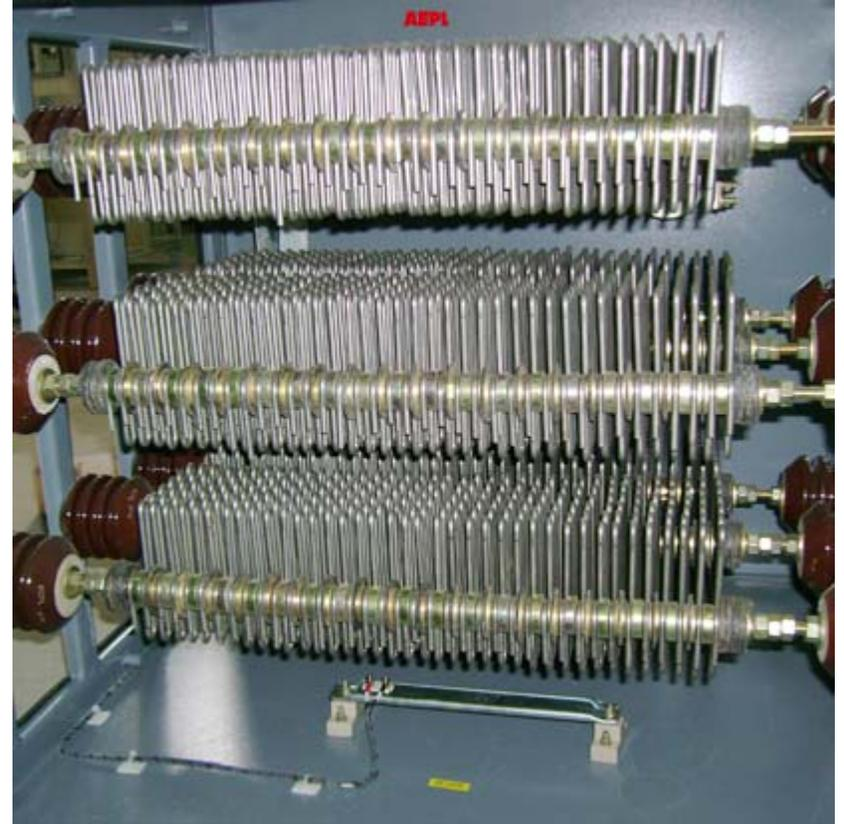
**Enclosures for resistors shall have openings to provide adequate ventilation, and shall be installed to prevent accumulation of combustible matter too near to hot parts**
